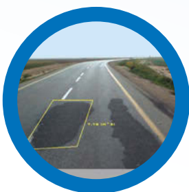
Area & Coordinates of Pothole Repair
